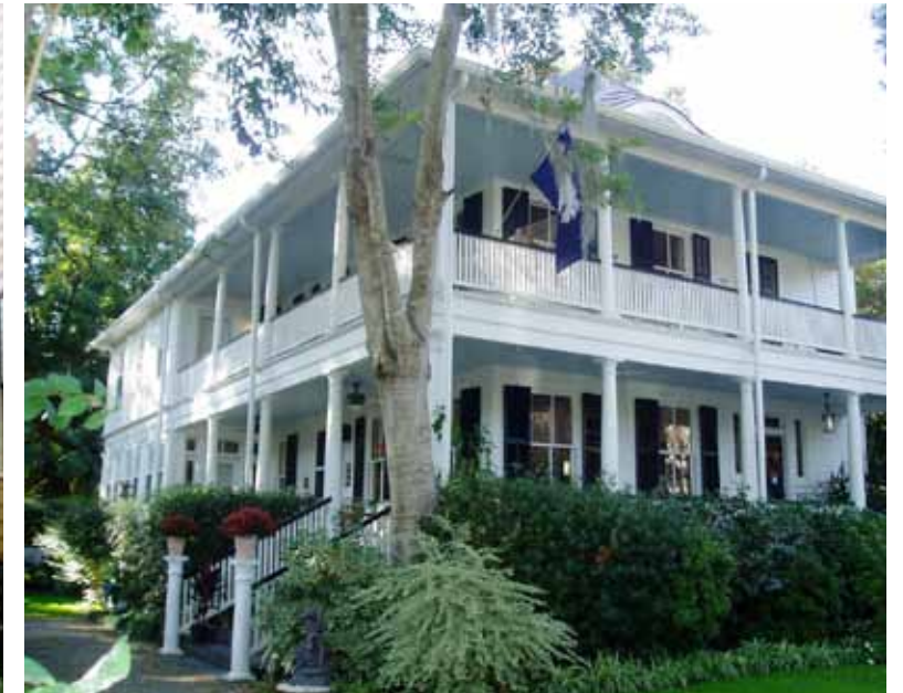
Typical wrap-around porch
