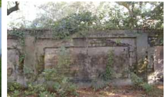
Aged brick wall
