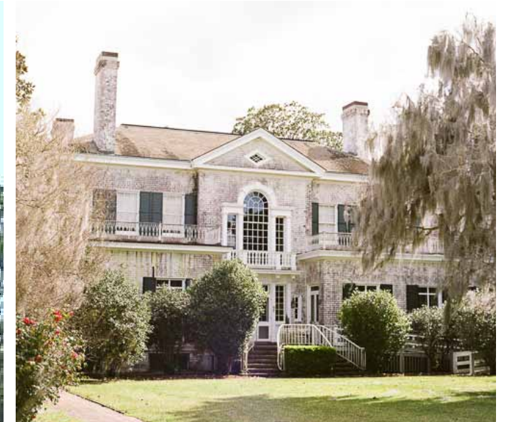
Brick Foundation and Chimneys
