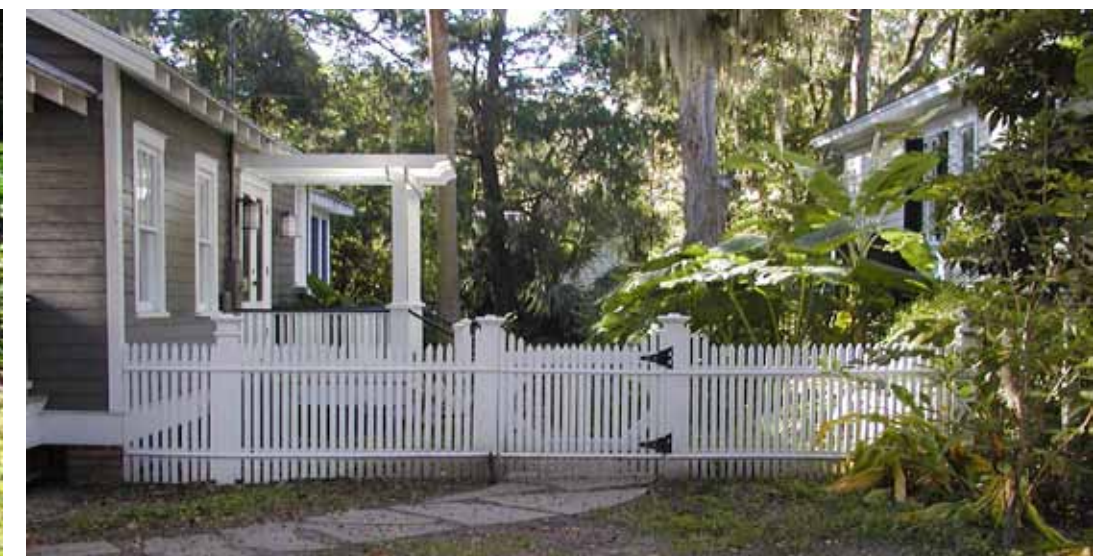
Wooden fence connects these two structures
