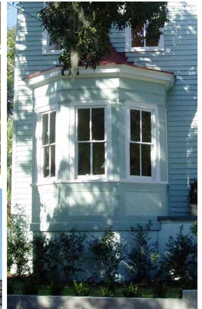
Bay window with proper execution
