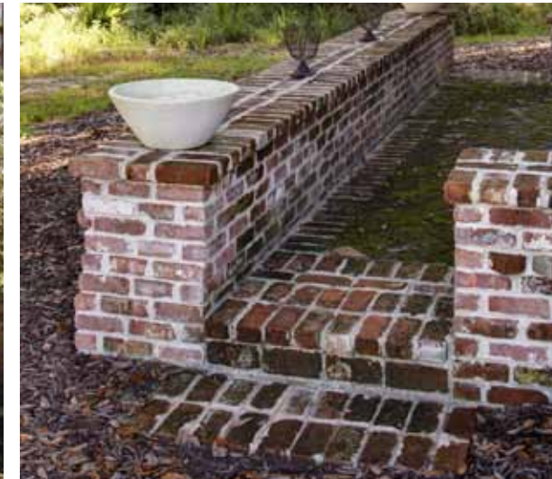
Low Brick Wall and patio
